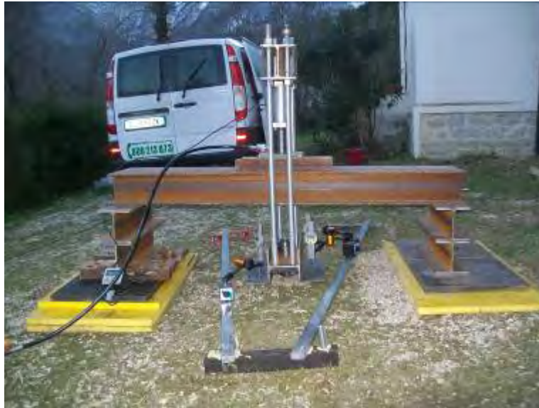
Figure 13: “Castle” apparatus for the execution of tension tests on RR micropiles in the sample site of Teramo, Italy.
