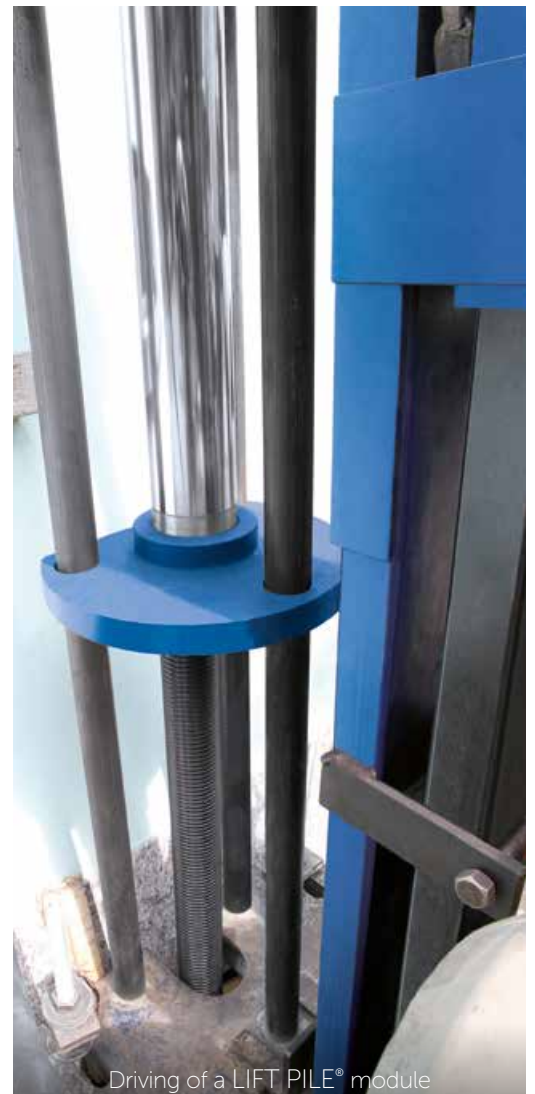
Driving of a LIFT PILE® module
